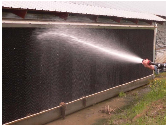
A gentle spray from a garden hose is best for rinsing pads. Cellulose pads are easily damaged with a high pressure washer.
